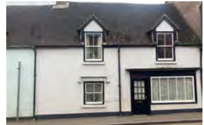
Figure 120: Positive example of a shop conversion into residential where the existing openings have been retained and now form part of the design of the property, Twyford.
