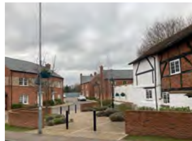
Figure 118: Local example of a recent small development within the conservation area that respects the massing and architectural styles of the neighbouring streets, High Street.
