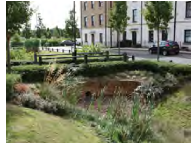
Figure 94: Example of swales integrated within the new development creating green links with the surrounding countryside, somewhere in UK.
