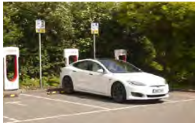
Figure 81: Example of electric vehicle charging points in a parking court.
