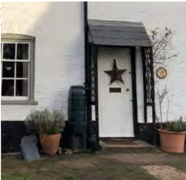
Figure 96: Examples of water butts used for rainwater harvesting in Reach, Cambridgeshire.
