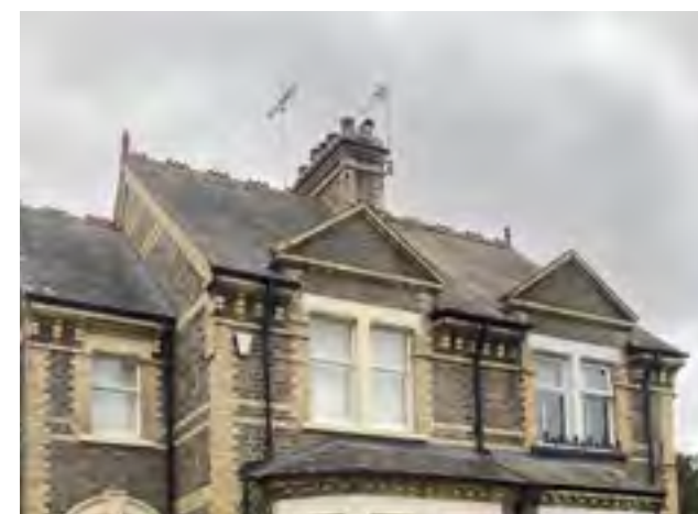
Figure 114: Local example, within the Station conservation area, of grey slate tiles on a gable roof with chimney.
