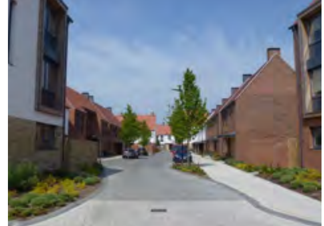
Figure 68: Tertiary street with inset parking bays alternating with trees on both sides in Dewenthorpe, York.
