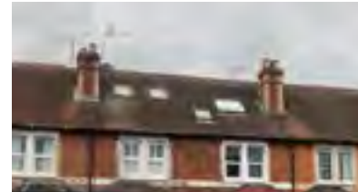
Gable roof with chimney stacks and rooflights
