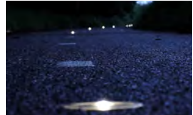
Figure 71: Example of a foot/cycle path which is lit by solar cat's-eye providing some light for pedestrian and cyclists without creating any disturbance to the nearby properties or unacceptable levels of light pollution.
