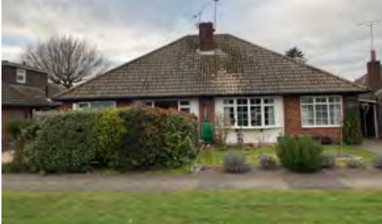
Figure 43: Buildings bordered with hedges, bushes and flower beds improve the environment whilst helping separate public from private space.
