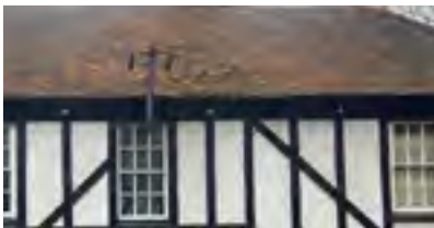
Half timbering technique infilled with off-white render
