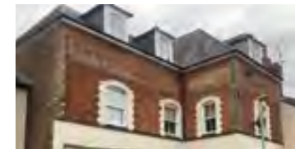
Hipped roof with hipped dormers
