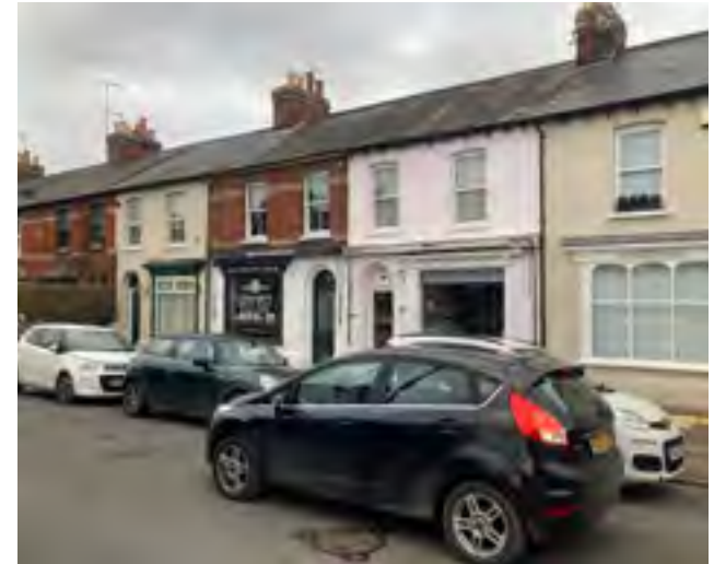
Figure 115: Local example of terraced housing within the Twyford Station Conservation Area.
