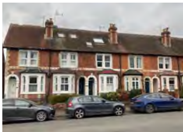
Figure 10: A row of Victorian style red brick terrace houses fronting onto Twyford Station, Station Road (Station Conservation Area)
