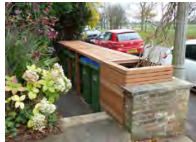
Figure 83: Example of wheelie bin storage for front gardens that include a green element to improve the aesthetics.
