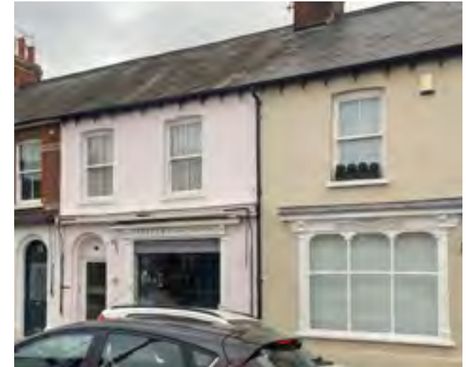
Figure 119: Positive example of a shop conversion into residential where the existing openings have been retained and now form part of the design of the property, Twyford.
